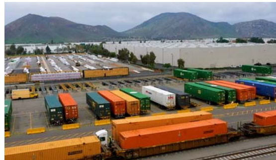
Inland Empire Intermodal Terminal Colton, California
